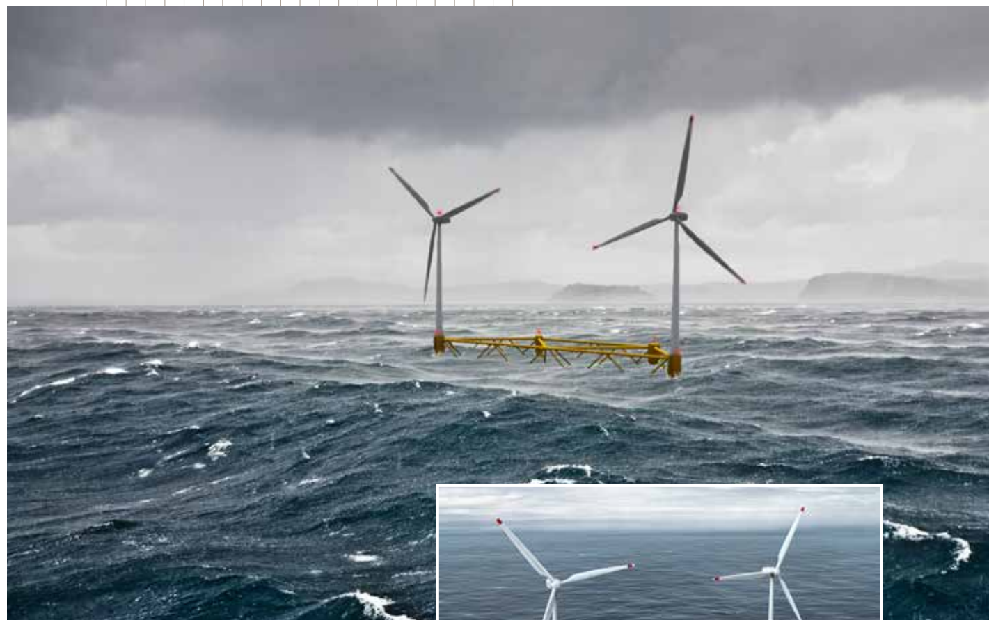
Hexicon floating wind turbine concept with two 5MW wind turbines on one floater
